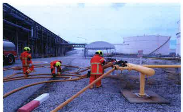
ERT connected 7 fire water hose from fire truck with foam connector of 60D255
